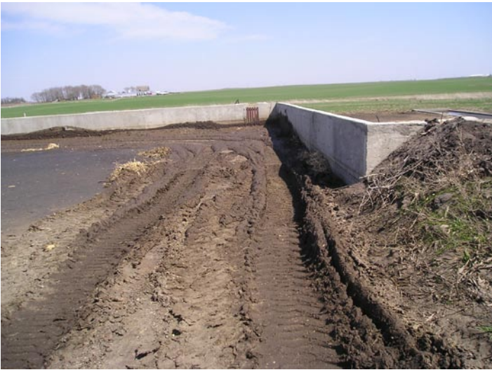
Solids settling walls & outlet. After catching runoff, solids are settled on the lot, and settled effluent is released.
